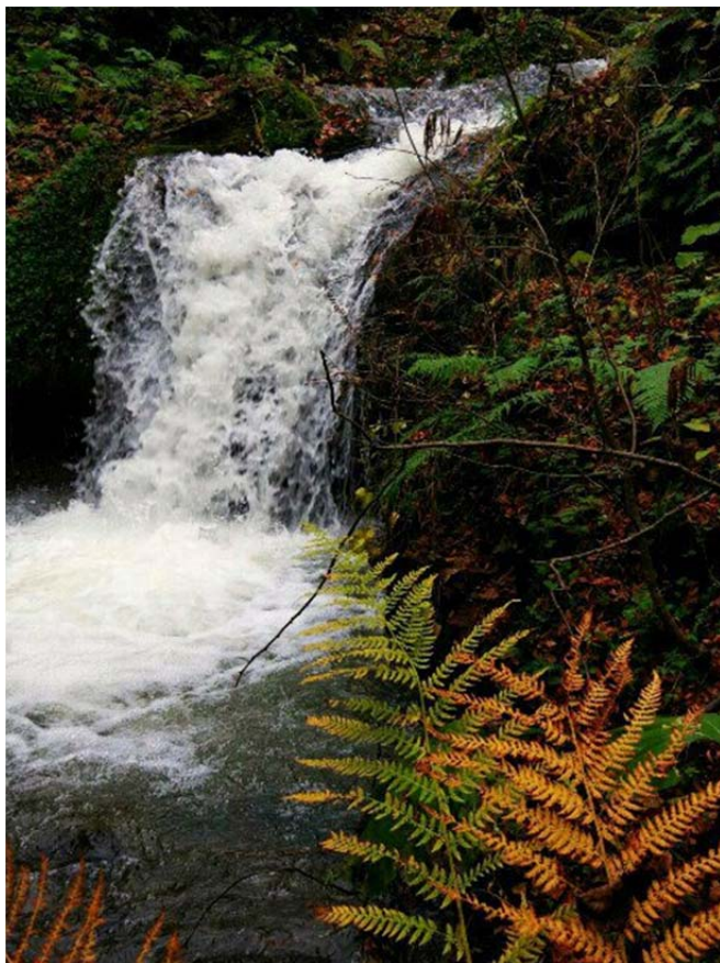
Figure 3a. 80 m upstream of power house SHPP Duboki Potok 2
