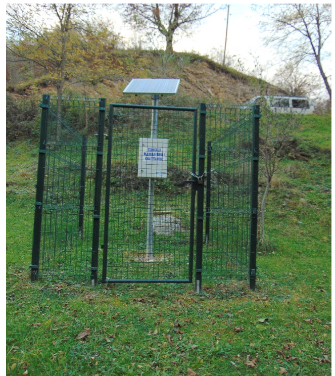
Figure 4b. Automatic hydrological and water quality station at SHPP Duboki potok 1
